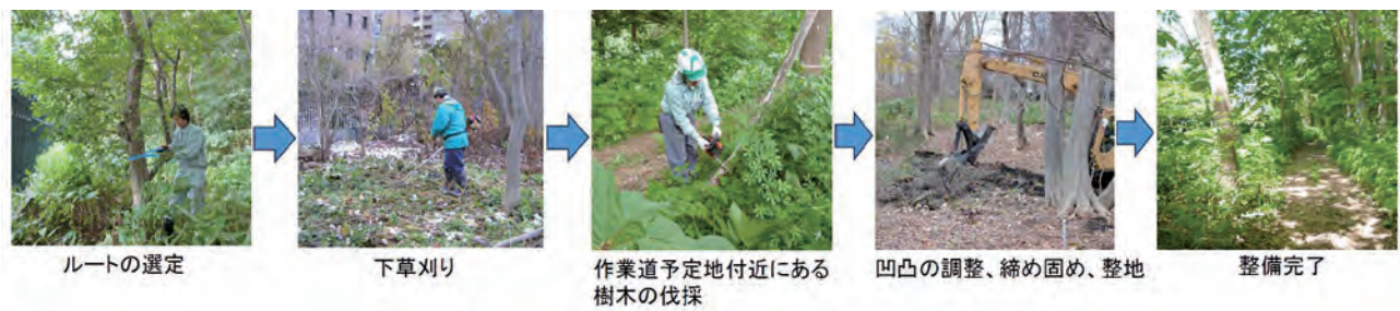
図4 作業道の新設。 Fig. 4 Construction of new work roads.
